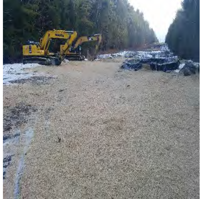
Fig 2: Str. 70 work area, note straw cover. Viewing east. (01-27-20).
