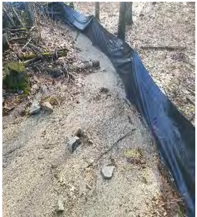
Fig 12: Sediment build-up on silt fence, runoff from rills at Getchell property/west side of the Bay. Viewing southeast. (01-27-20)
