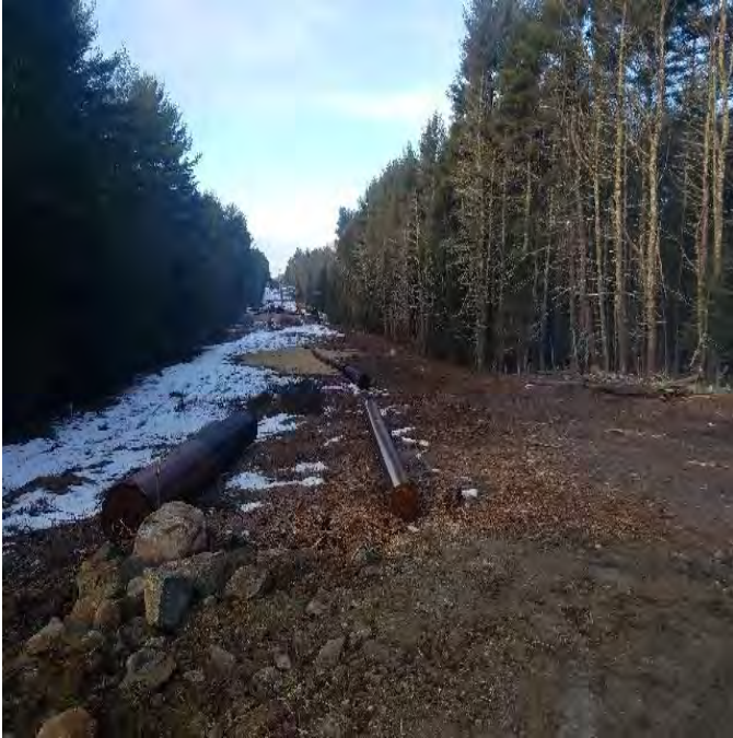
Fig 1: Access to Str. 71. Viewing west (01-27-20).
